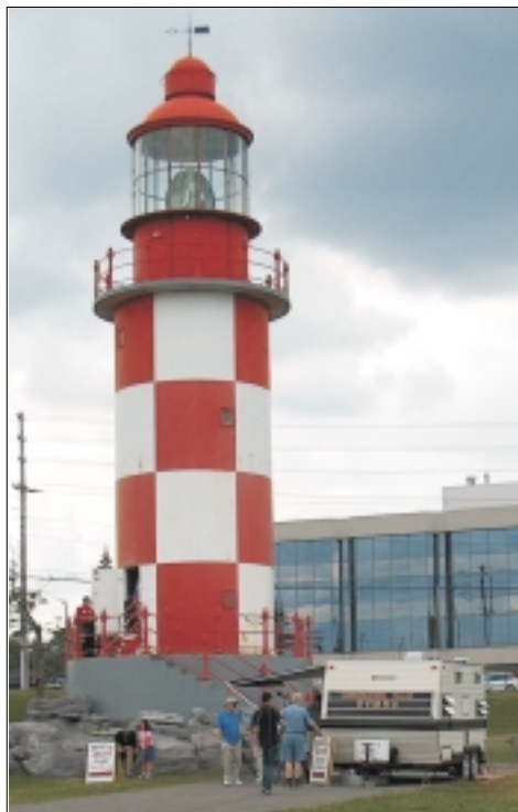
CMST Lighthouse and OVMRC Trailer.
